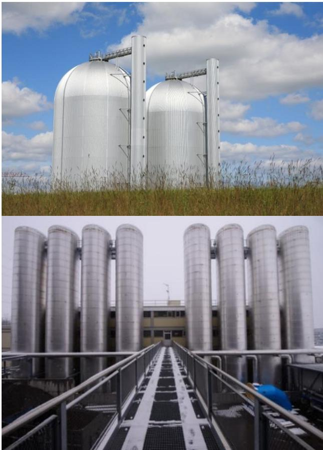
**Abbildung 4-2: Avenore TTES 2 x 24'000m<sup>3</sup>, max. 120 °C / Buchs, 8 x 200 m<sup>3</sup>, max. 150 °C**
